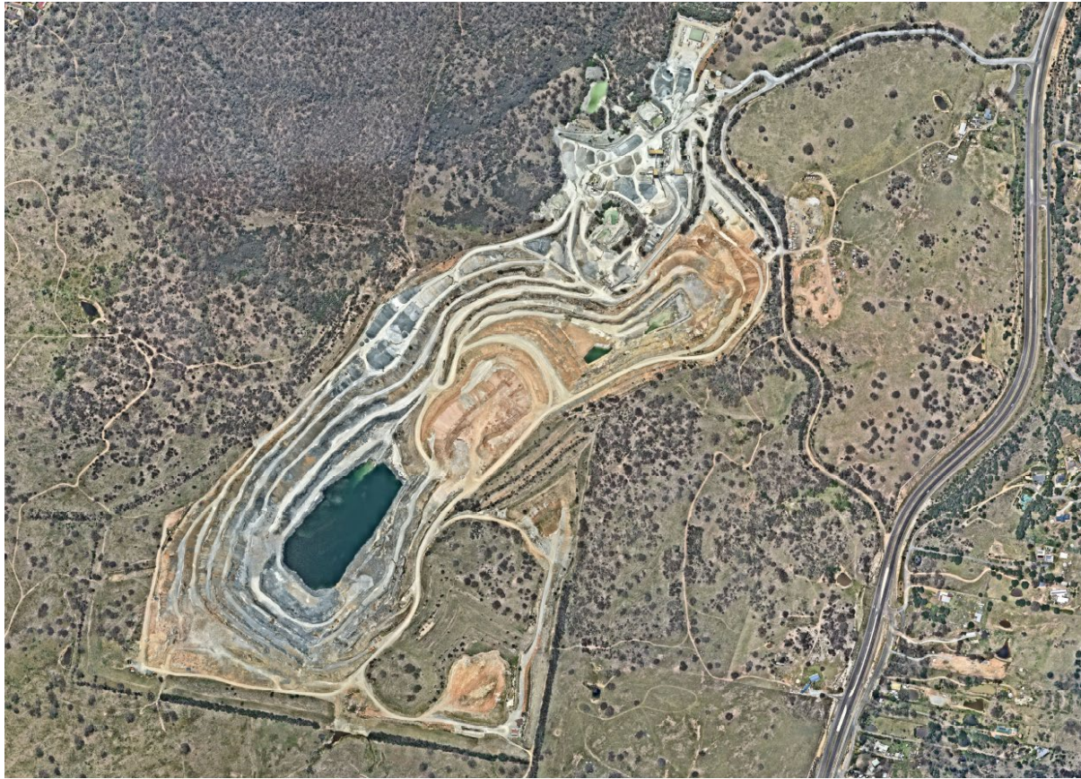
Figure 2: Aerial view of the Cooma Road Quarry (source nearmaps 2023)
